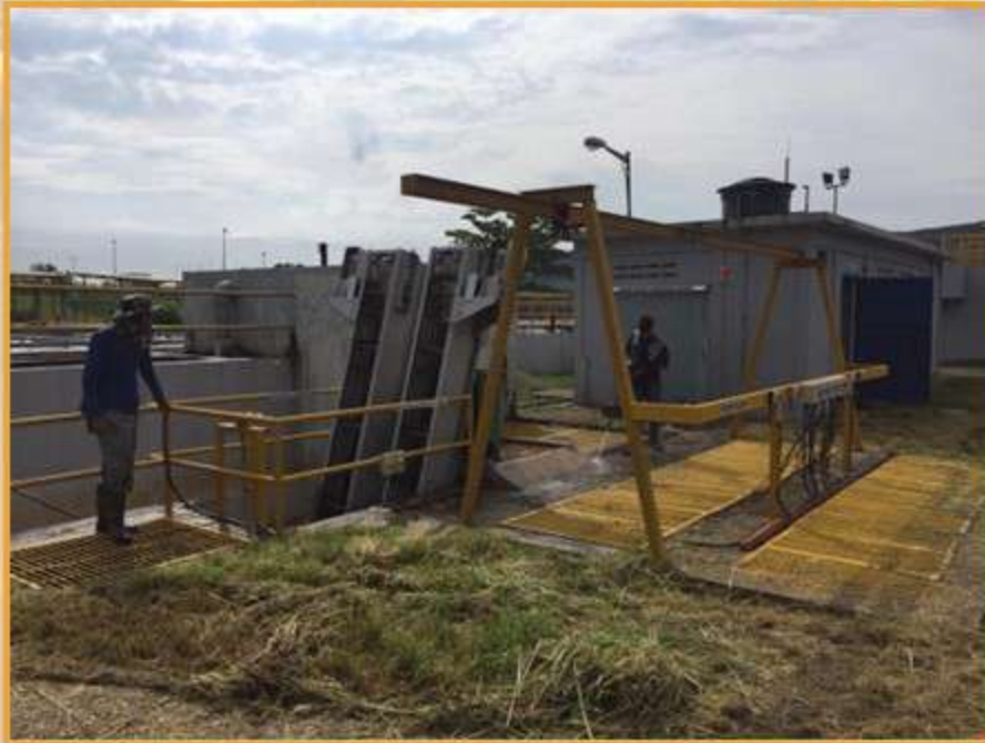
Kerja-kerja Servis Coarse Mechanical Screen
